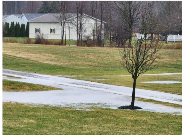
Apr 2025 — stormwater sheeting across yard & driveway.
