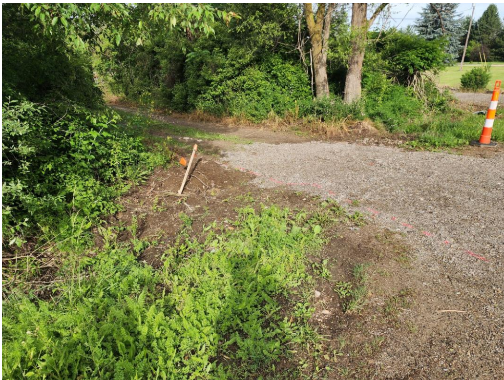
Exhibit E3 — Jun 15, 2026 (AFTER): the approach at parcel 10-10-400-023 where the driveway culvert was removed; survey stakes / flags present.
