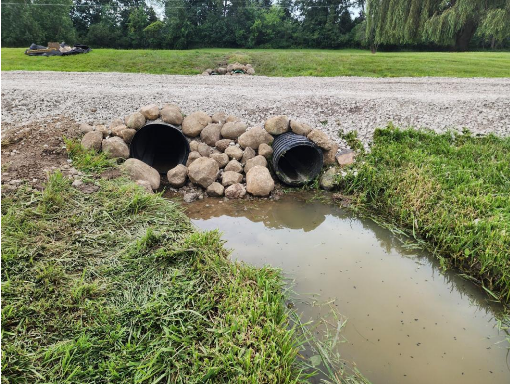
Exhibit C1 — Aug 5, 2024: TWO culverts installed under the driveway at the pond (doubled capacity) to try to carry the flow.
