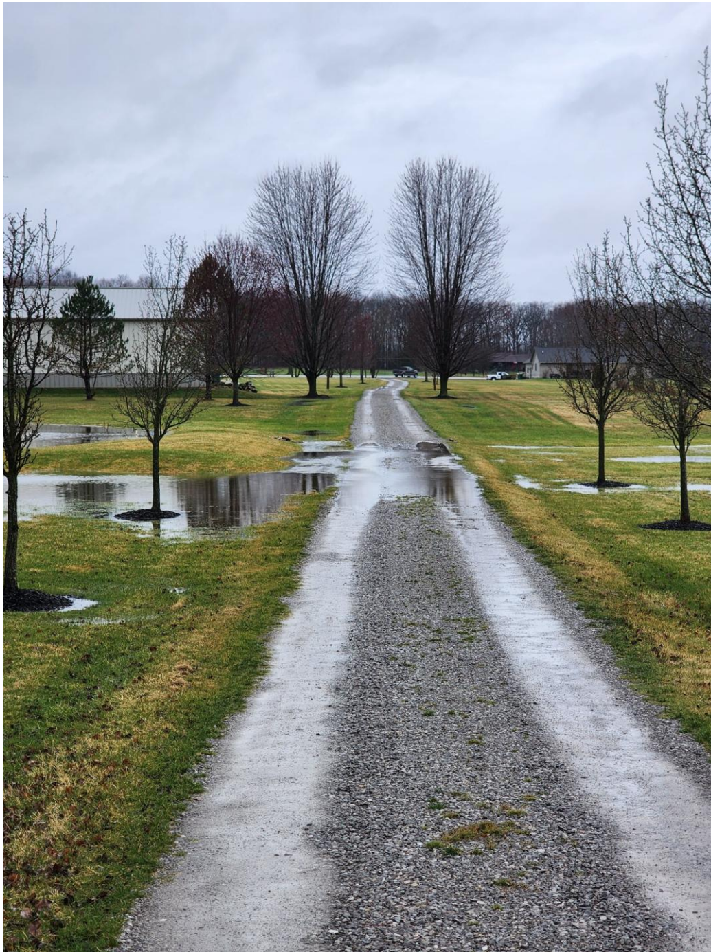
Exhibit B2 — Apr 2, 2025: the drainage line running full across the property.
