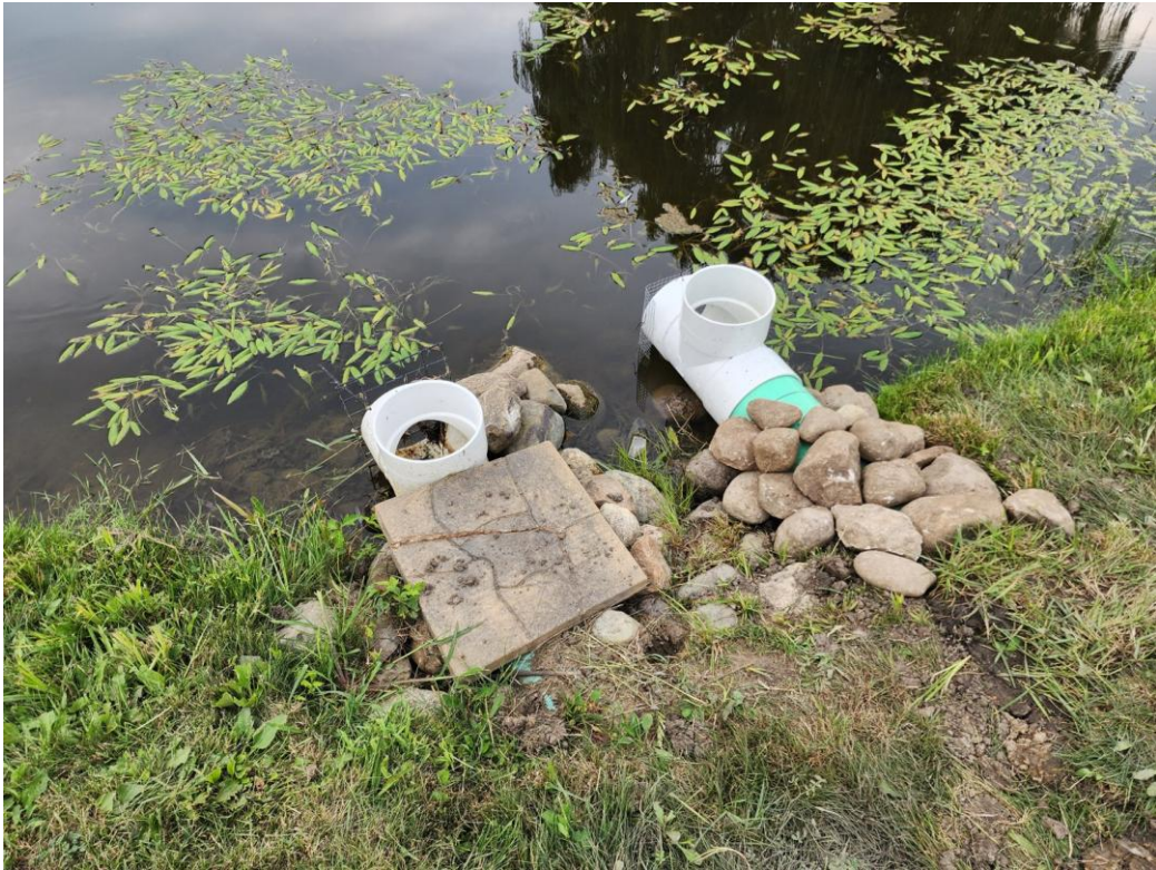
Exhibit C2 — Aug 5, 2024: the pond outlet structure — two outlets where there was effectively one before.
