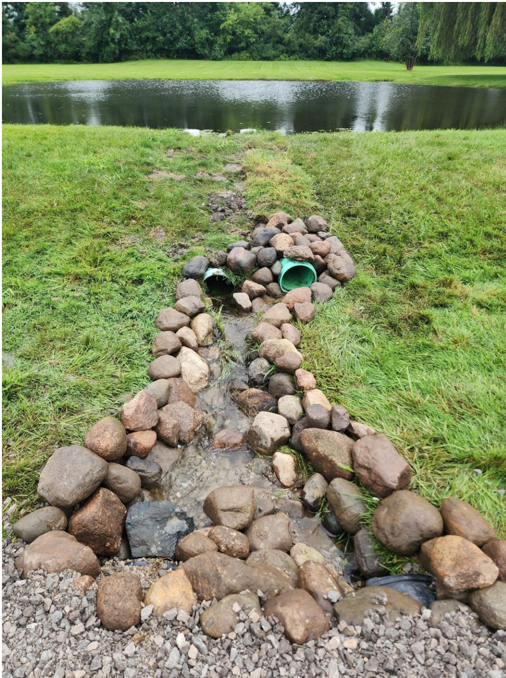
Exhibit C3 — Aug 6, 2024: rock-lined channel the owner built to manage the concentrated flow.
