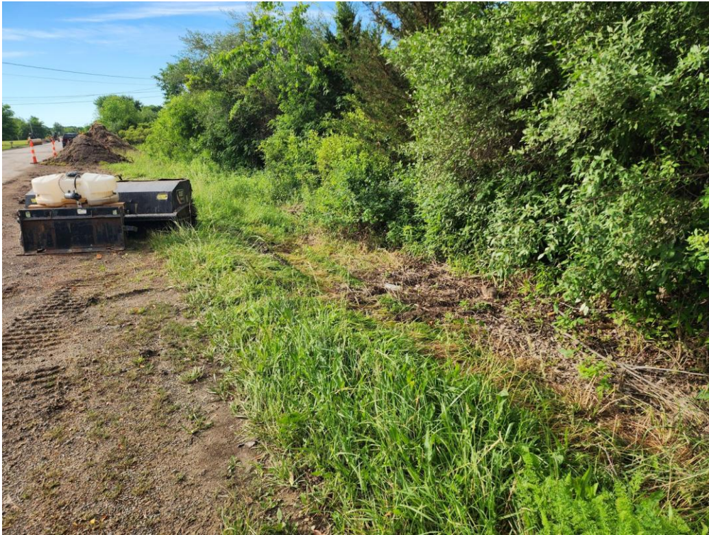
Exhibit E4 — Jun 15, 2026 (AFTER): the west-side ditch left overgrown and un-re-ditched alongside the construction equipment.
